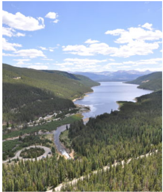
The 5.5 mile Boustead Tunnel (bottom middle) transports water from the Fryingpan River drainage underneath the Continental Divide into the Arkansas River by way of Turquoise Lake (top right) as part of the Fryingpan-Arkansas project. Photo courtesy of Klambpatten (with the Bureau of Reclamation).
